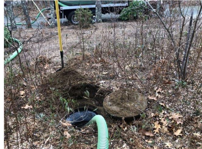
Septic Tank being pumped out
